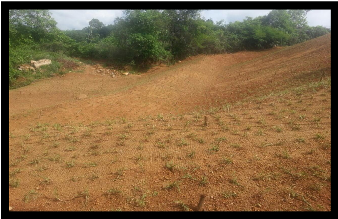
Over burden managed within the site
