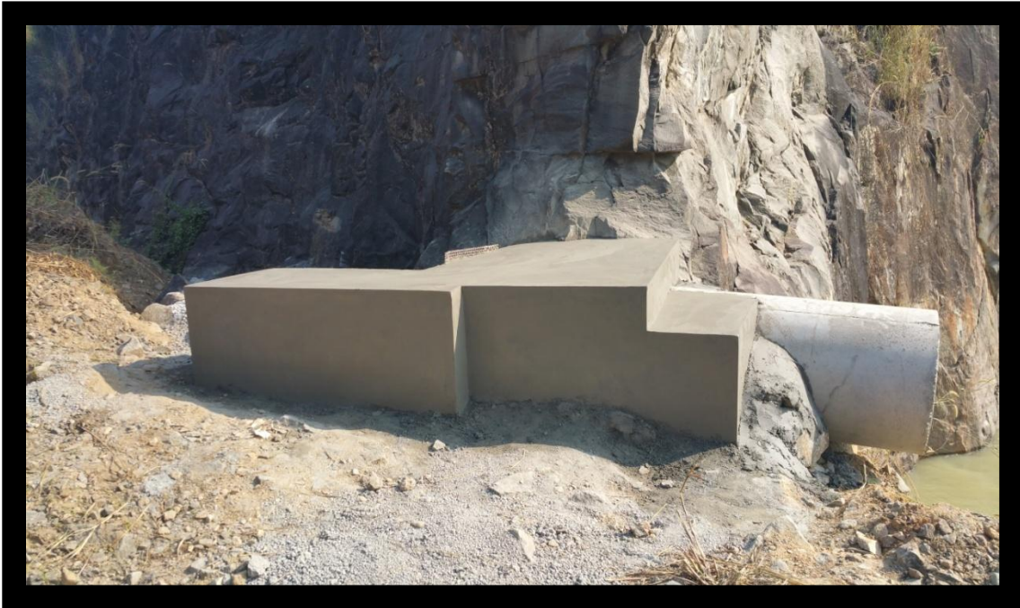
Drainage in the project site
