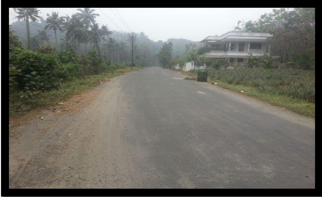
Tarred road to the crusher unit
