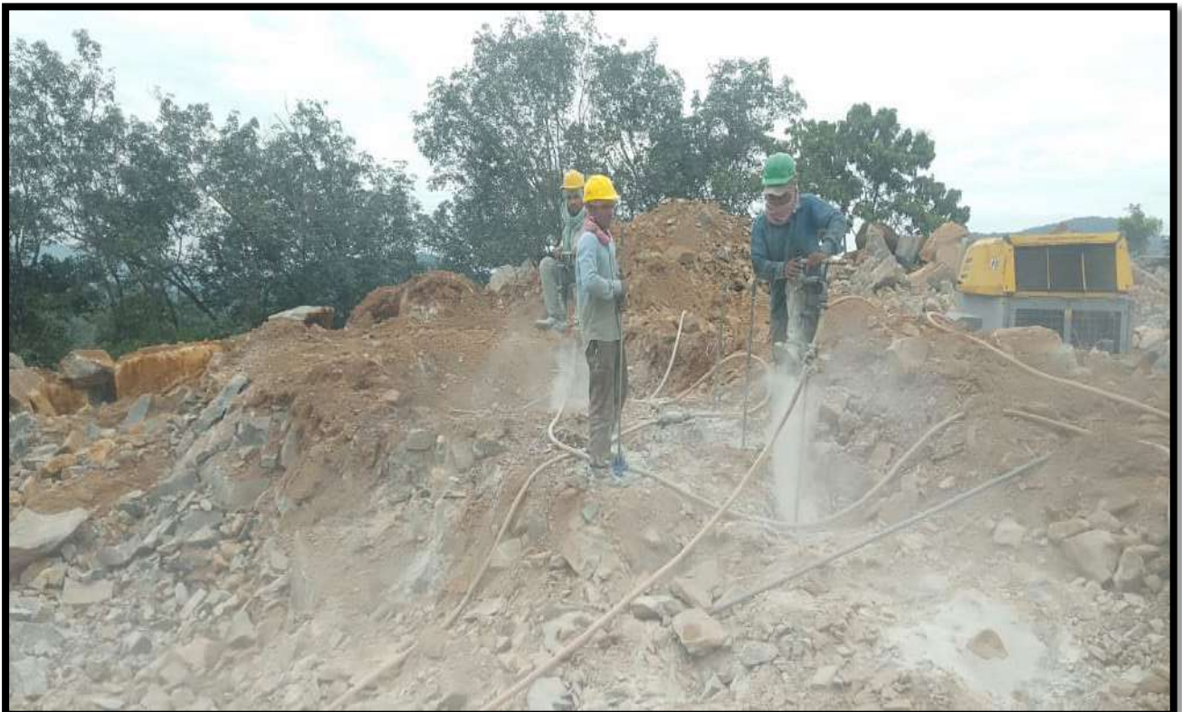
Labors with PPE
