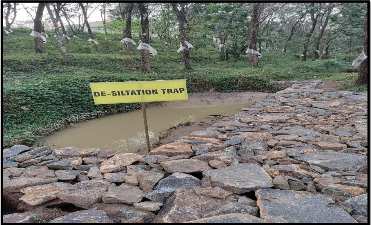
Clarifiers Plate No. 18
