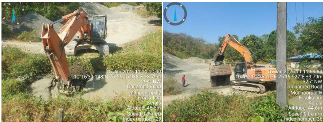
Geo tagged photograph of de silting process
