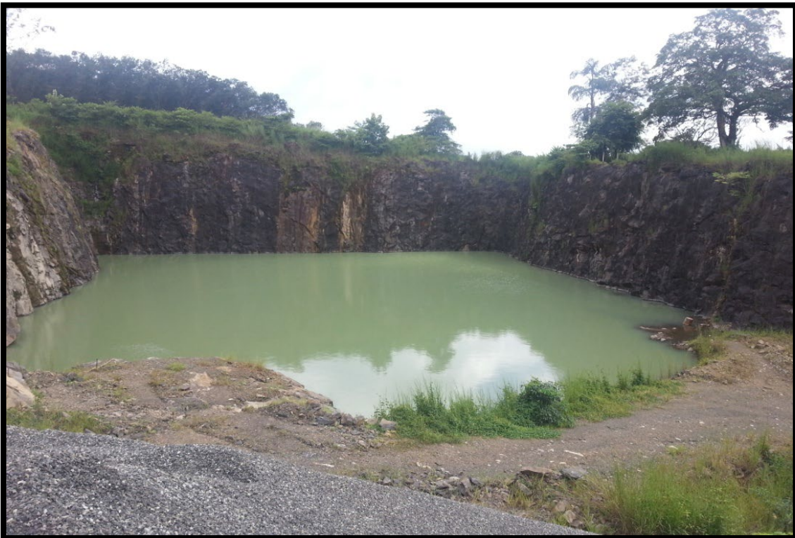
Rain water collection pond exist in the project site
