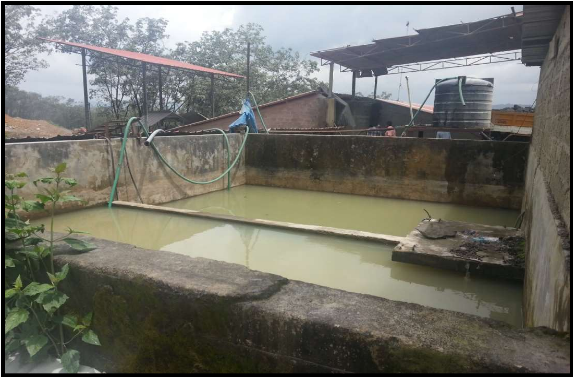
Rain water collection tank
